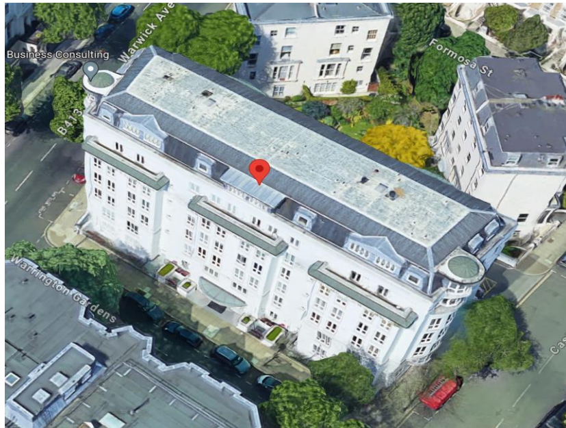
Figure 1: Overview of Southeast elevation (Main Entrance)
